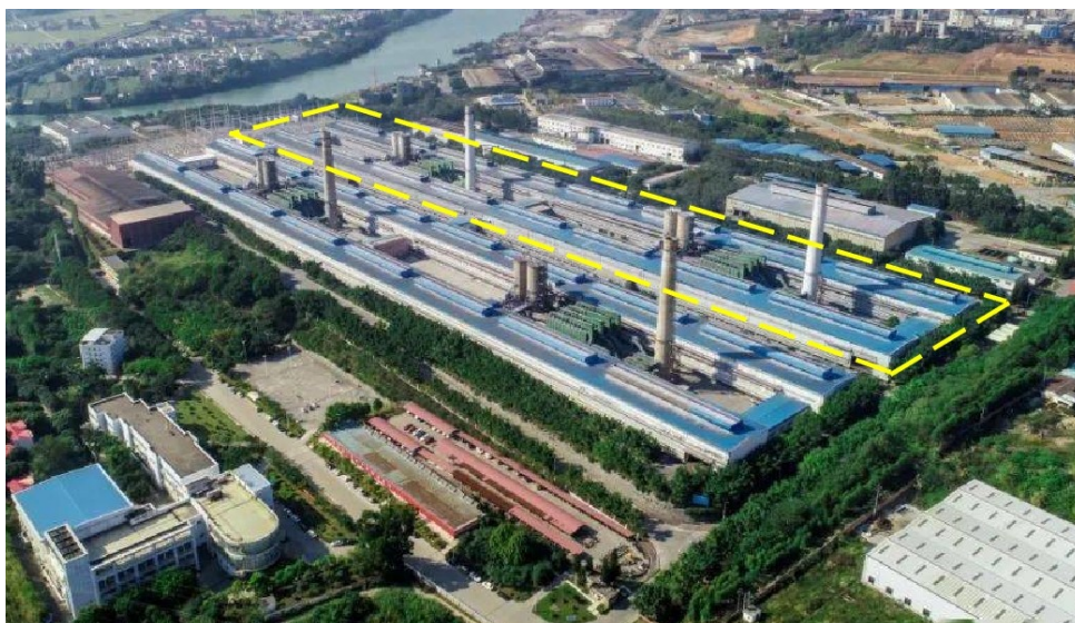
Figure 1. Aerial view of the 240 kA potline.
